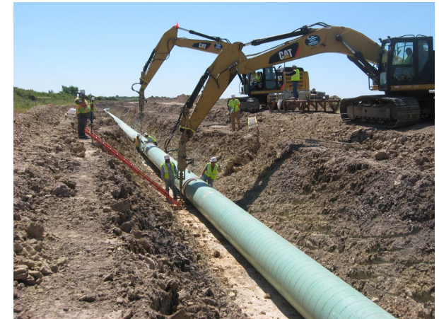
FERC ditch showing extra material excavated
