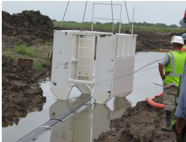
Portable trench box being used with divers
