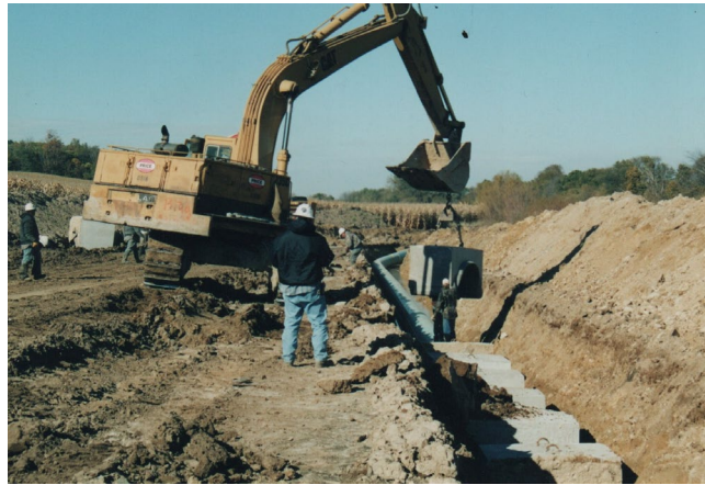
Concrete weights being installed on 36" pipeline
