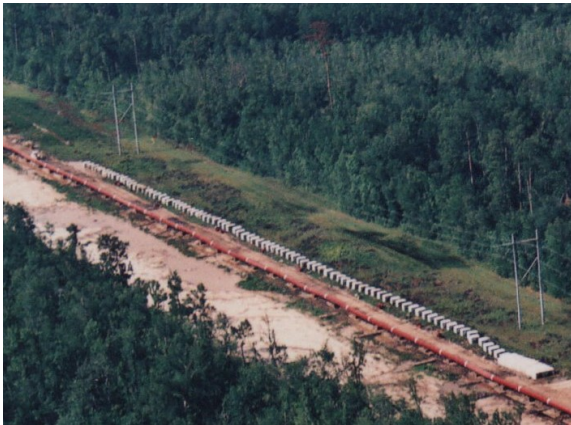
Concrete weights on right of way ready to be installed
